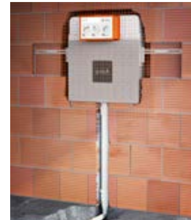
Concealed cistern suitable for squatting pans.
